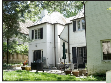
Covered Porch Addition Clayton, MO
