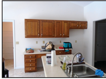
Glencoe Kitchen Remodel
