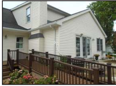
Glencoe Back Porch Addition
